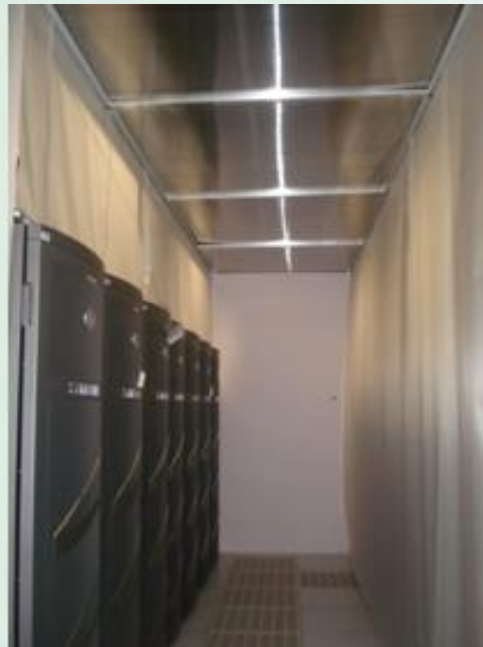
Wide cold aisle with a single row
