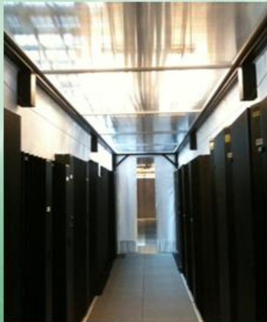
Wide cold aisle with 2 rows of racks
