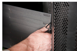
Place the panel in the required position and align the clips with 19" mounting holes
