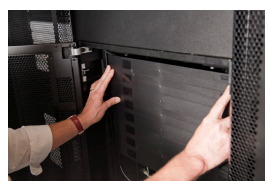
Insert the adjusted panel to fill the remaining open rack space.
