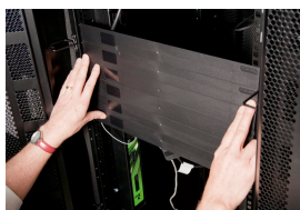
Push the clips firmly into position on each side
